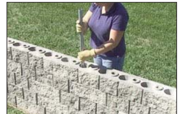
Remove top blocks as you drive the pipe into the ground.
